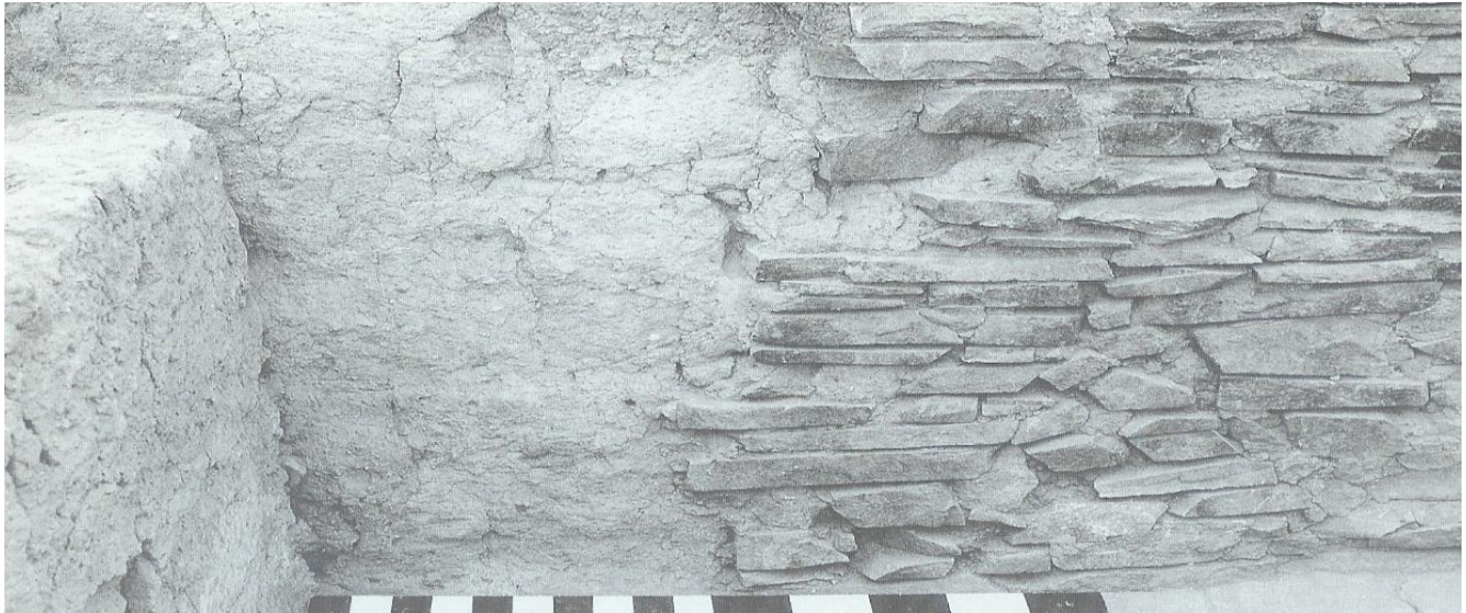
Figure 14. Adobe and masonry wall abutment in room 11-5, illustrating the shift from masonry to adobe construction.
